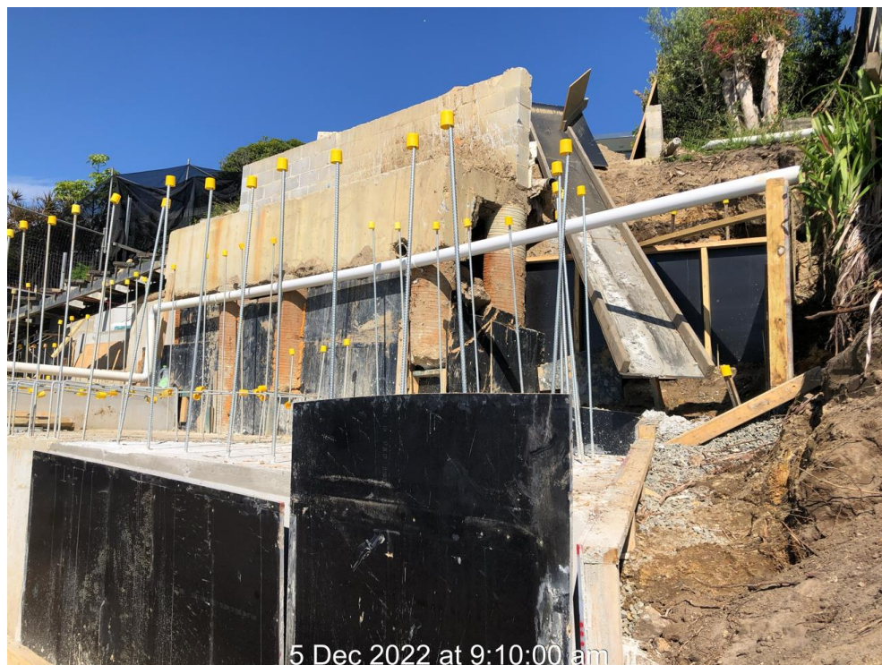
Figure 11: Photo of subject site on 5/12/2022 noting waffle pod footings on northern portion of site and starter bars
